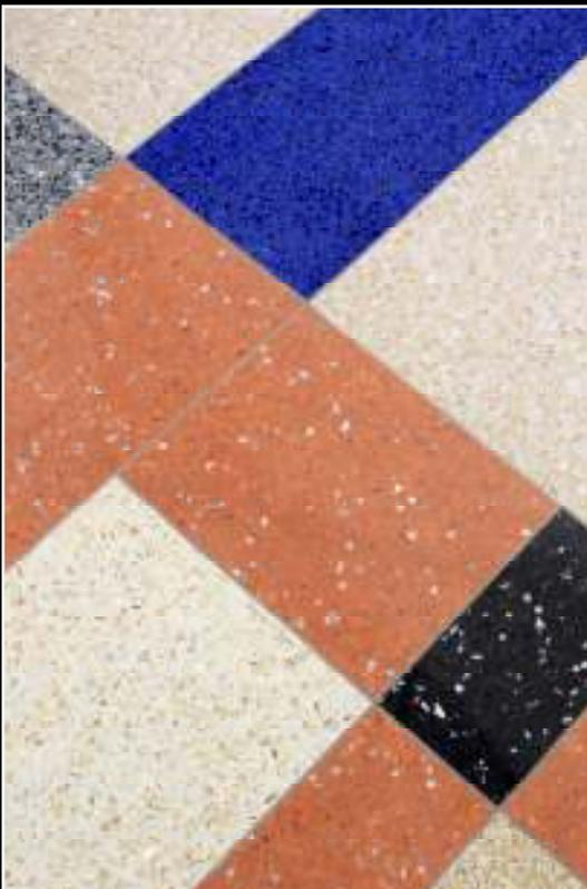
Terrazzo is a composition material that is poured in place. It consists of marble aggregate with either a cementitious or epoxy binder. It is poured, cured, ground, and then polished.
